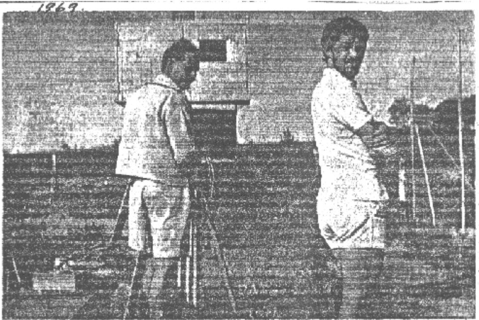
The fitting of lights at R.I.T.A. courts at the Cleveland Showgrounds is awaited with much interest by many tennis fans. Here the electrician attends to a mass of wiring of the first light to be installed; watched by tennis player, Robert Kees. Night tennis — just the thing for winter.
